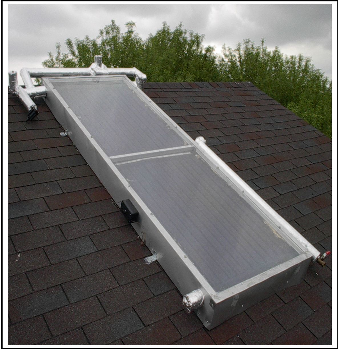
Roof Mounted Hot Water Collector (Rated 1.4KWh)
